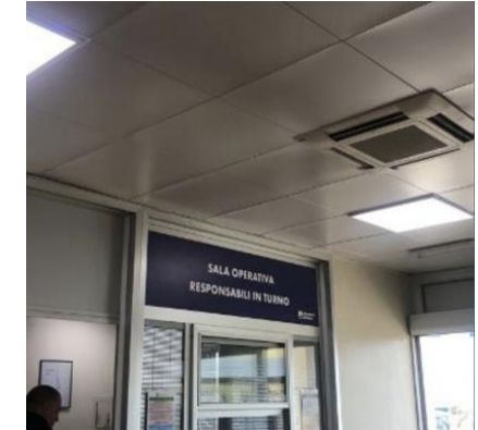
ADR- Rome Fiumicino Airport Emergency Hospital
